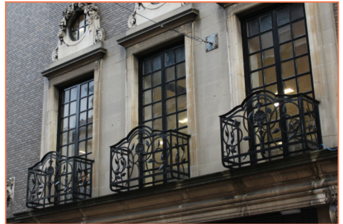
Ironwork to first floor balconies
