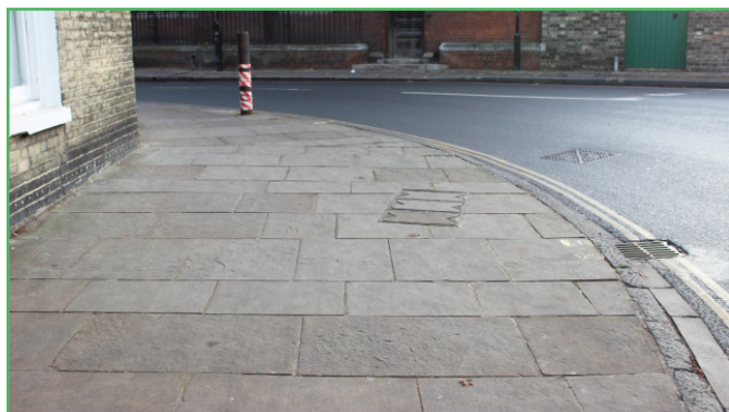
York stone paving and granite kerbs
