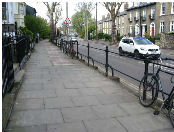
Raised pavement in Maids Causeway
