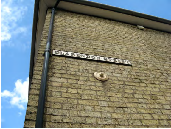
Cast iron nameplate on No. 40 Clarendon Street
