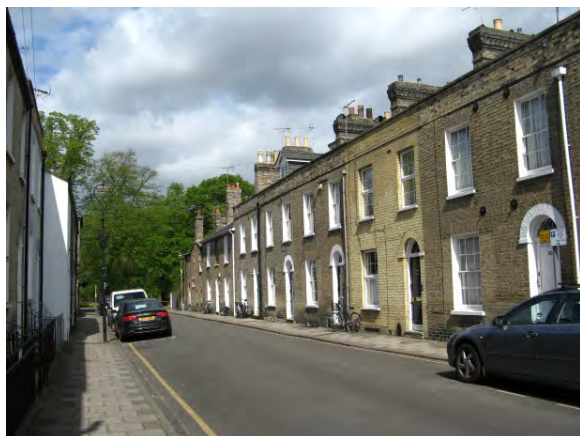
Nos. 2-10 (even) Earl Street
