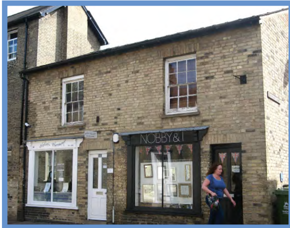
Shopfronts to Nos. 13 and 14 Fair Street
