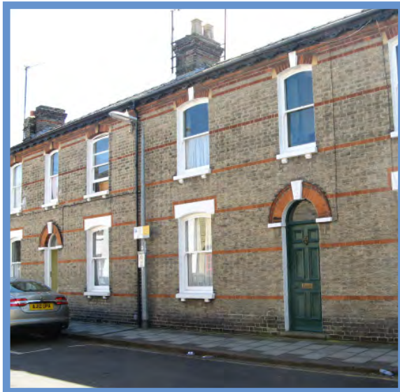
North side of John Street
