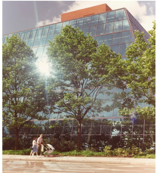
Figure 41: Solar dazzle reflected from a glazed façade
