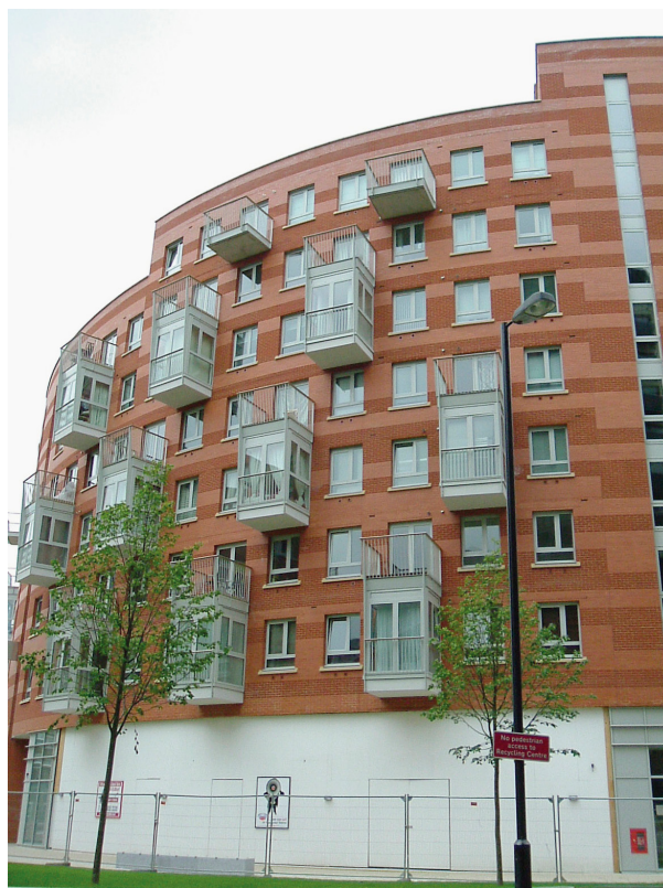
Figure 13: This North London development (architects CZWG) has staggered balconies to minimise obstruction to living rooms. Where a balcony is above a living room the obstructed area has been modified to form an unobstructed bay window.
