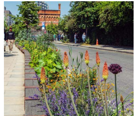
Use of rain gardens as a buffer between vehicle and pedestrian routes. Camley Street, London, LDA Design
