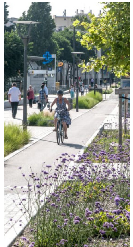
Wide cycle lanes along SuDS planting Avenues Mermoz et Pinel, Gautier+Conquet Architects, France
