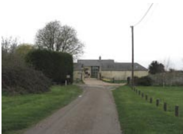
Track to Alwyns Barn
