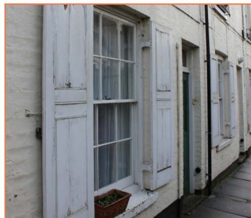
External shutters at ground floor
