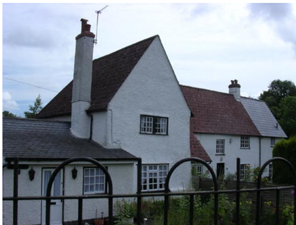
Nos 82 & 84 Main Road
