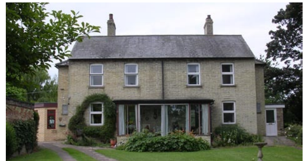
Nos 15 & 17 (Rectory Cottages) Church Walk
