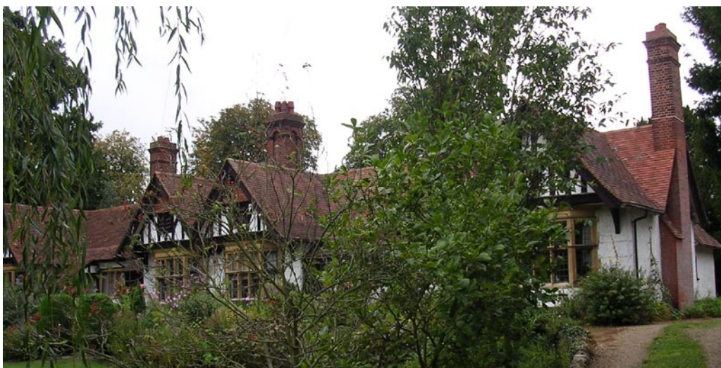
Almshouses at 2-8 Church St
