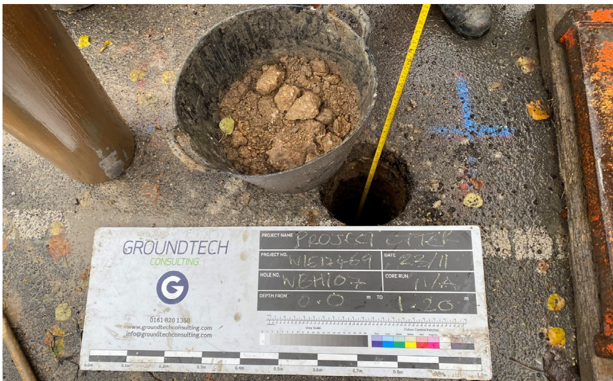
Photograph 12 – WBH107 Inspection pit
