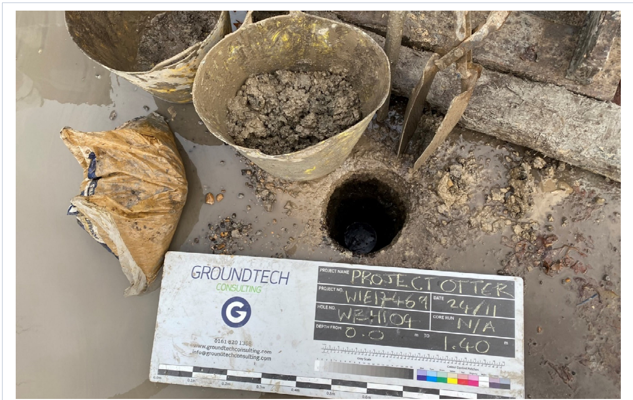
Photograph 9 – WBH104 inspection pit
