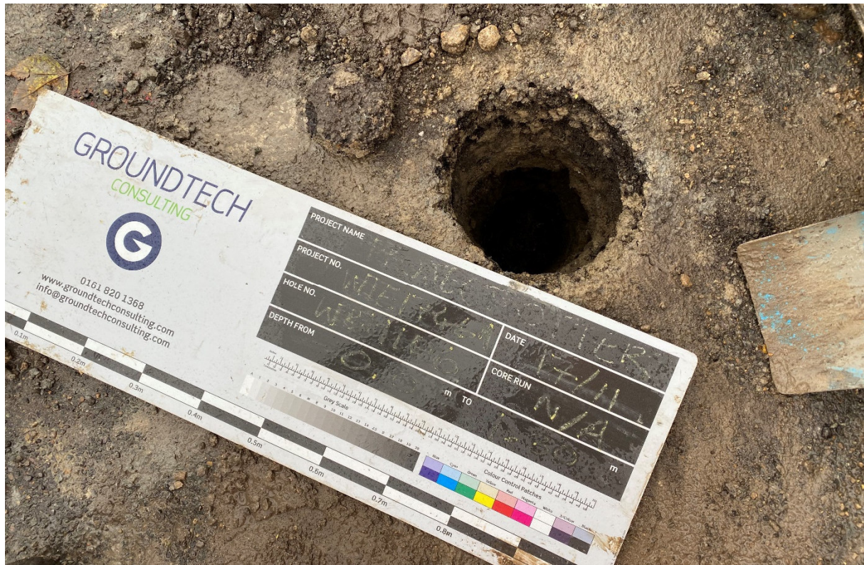
Photograph 11 – WBH106 inspection pit
