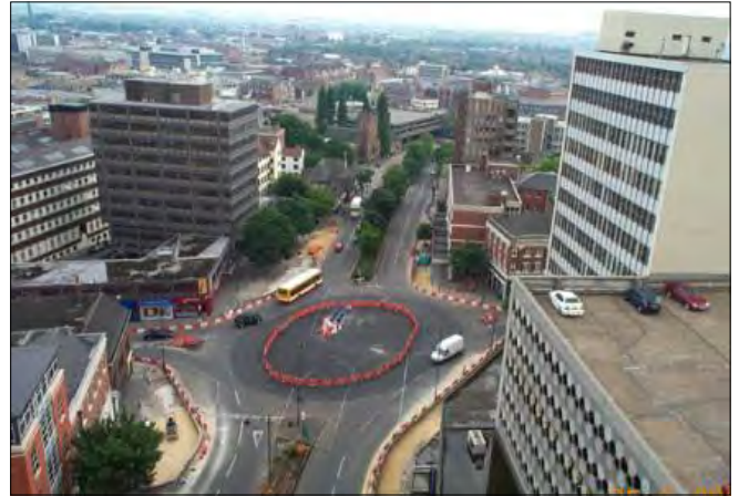
Figure 46: Filling in the subways with concrete
