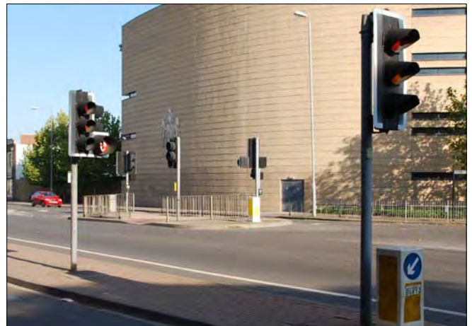
Figure 13: Pedestrian guardrails present barriers to movement
