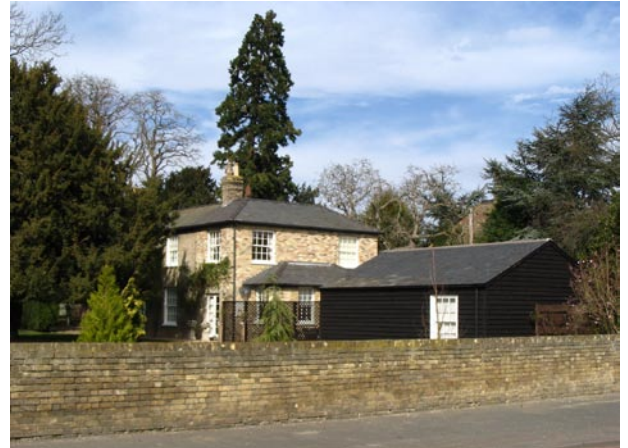
The rear of the Old Rectory
