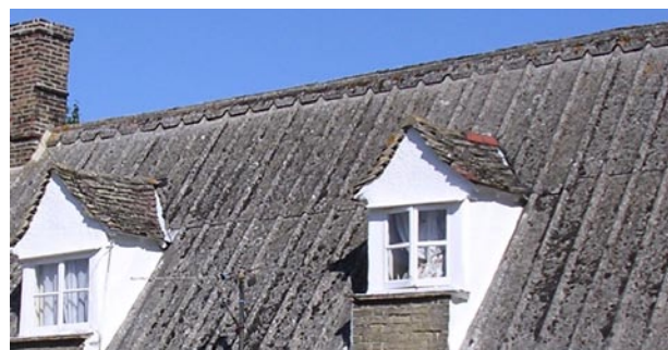
Example of former thatch roof now covered in asbestos sheet
