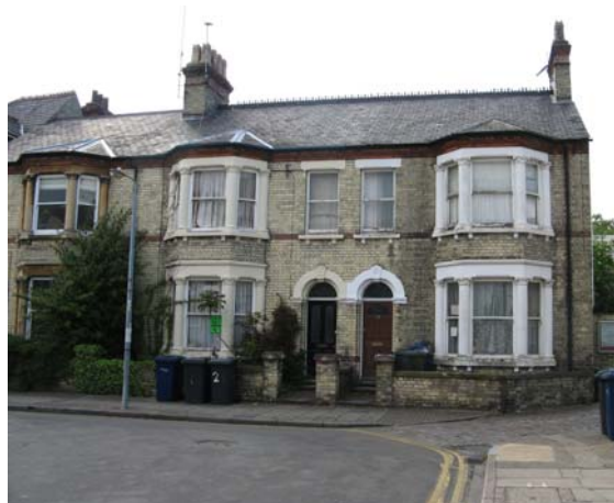
Nos. 19, 21 and 23 Willis Road
