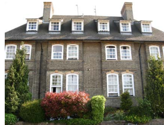
Nos. 1 and 2 Wollaston Road
