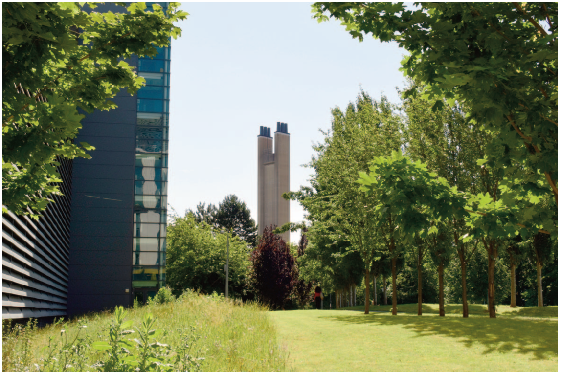
Image 6: Addenbrooke's Hospital incinerator chimney
