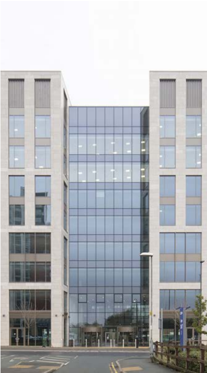
Plant screen integrated into glazing pattern Wellington Place, Leeds, Sheppard Robson
