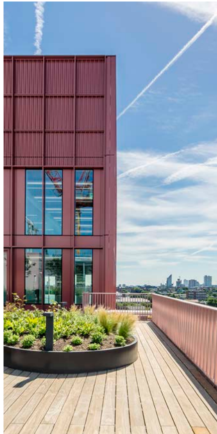
Architecturally integrated plant screen. R7 Kings Cross, London, Morris + Company
