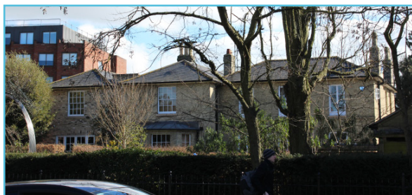
No. 2 Gresham Road hidden within garden
