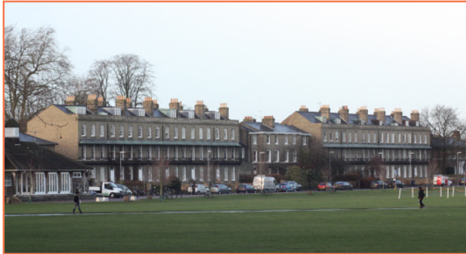
Views to Park Terrace
