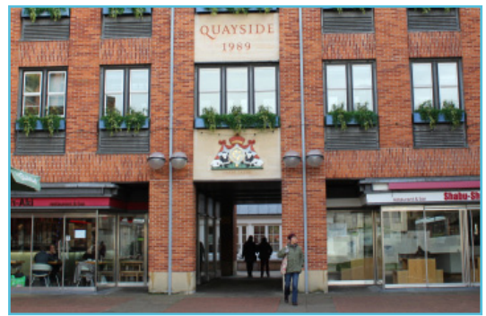
Tunnels to enclosed courts
