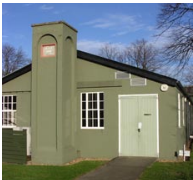
Building 80 Carpenters Shop and Dope Shop
