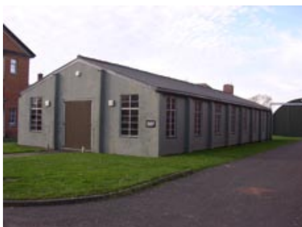
Building 286 and Building 287
