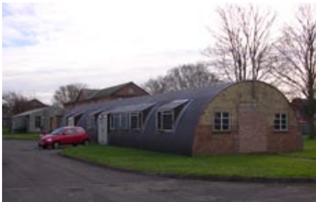
Building 285 NAAFI from north
