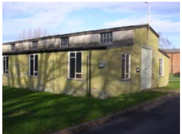
Building 147 Barrack Block of 1918
