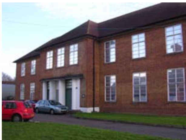
Building 215 Dining Room from north
