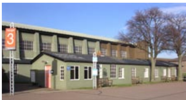
Building 89 Flight Office with Building 84 behind
