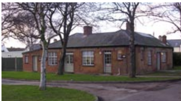
Building 48 works maintenance yard and building
