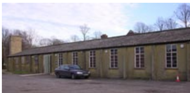
Building 288 from south and Building 288 from Parade Ground
