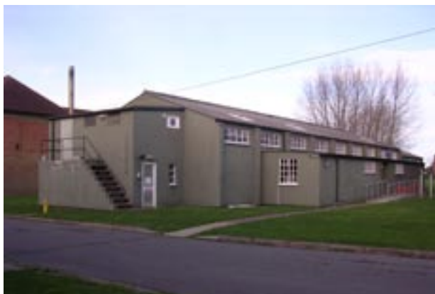
Building 207 Gymnasium and Chapel
