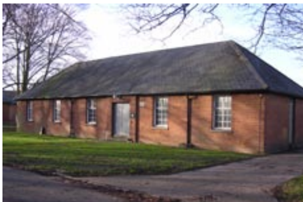
Building 11 Barrack Block for airman pilots
