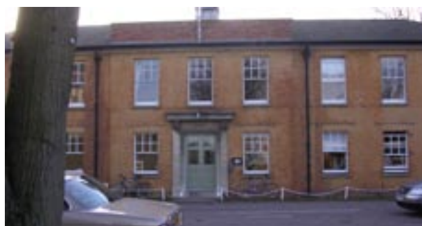
Building 61 Station Offices
