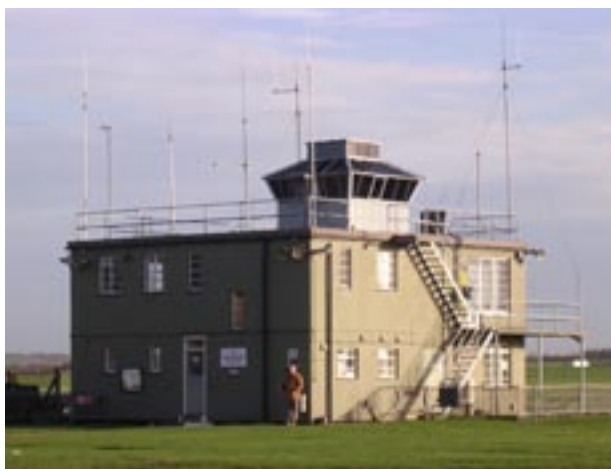
Building 209 Control Tower/Watch Office
