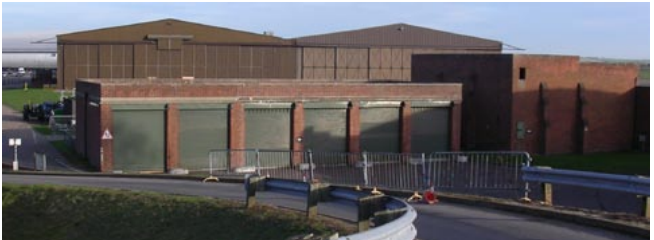
Building 70 with Hangar 2 behind
