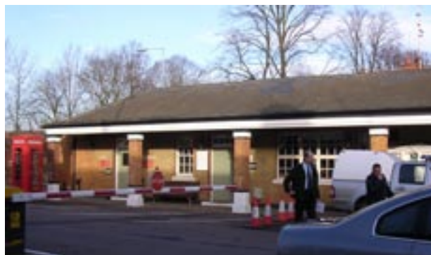
Building 62 Guard-house and K6 telephone kiosk
