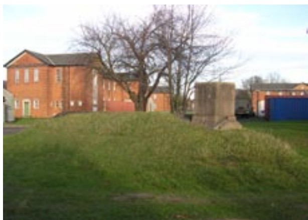
Building 9 Airmen's Barracks and air-raid shelter between Buildings 8 and 13
