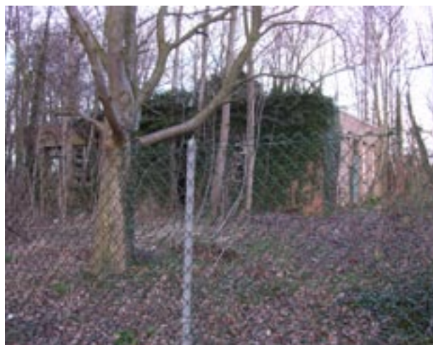
Building 91 W/T and R/T Transmitting Building
