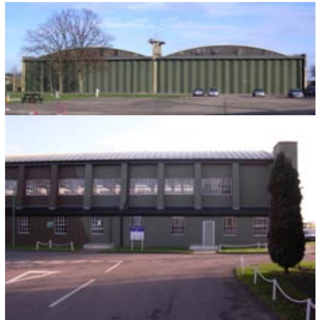
Building 84 1917 Hangar from the west and Building 79 1917 Hangar from the north
