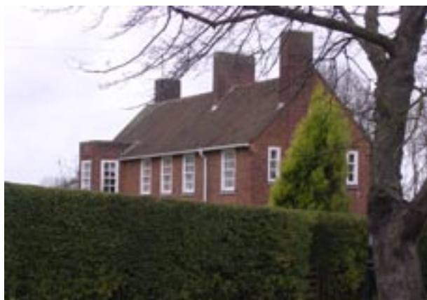
No 30 Ledo Road from the south east
