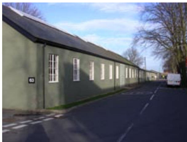
Building 63 Technical Stores with Building 66 beyond
