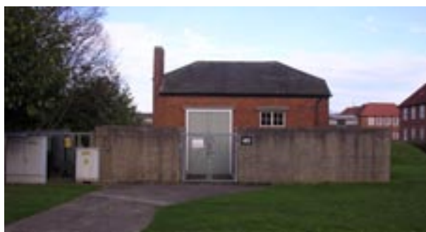
Building 40 Stand-by-Set House
