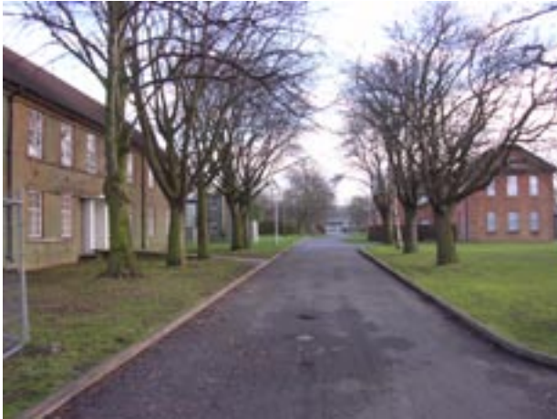
View looking south with Building 213 on left and Building 7 on right
