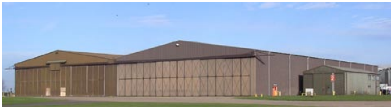
Hangar 2 North and South (type T2) from the west.
