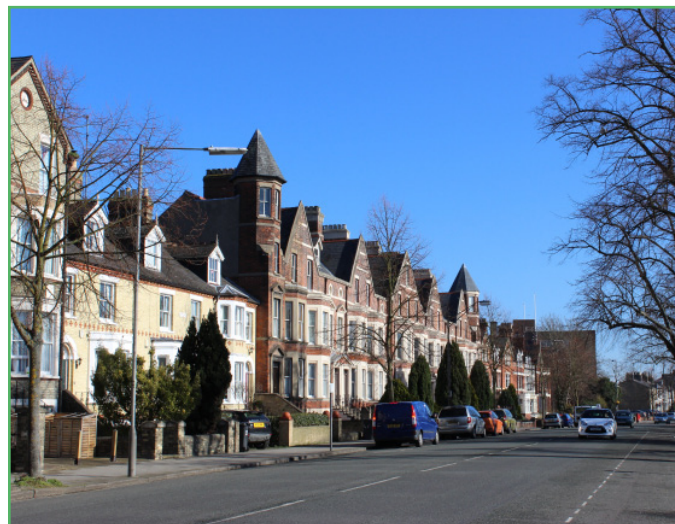
Detailing to brick houses
