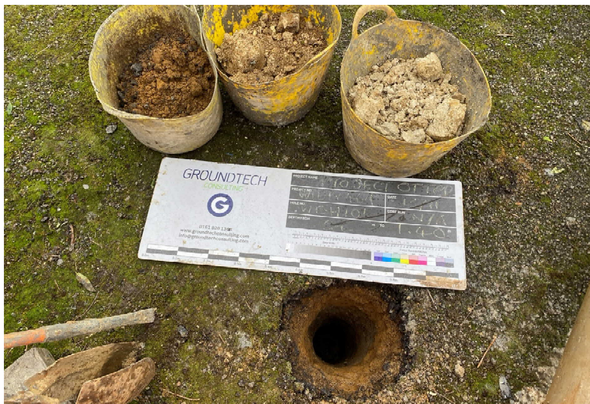
Photograph 5 – WBH101 Inspection pit.
