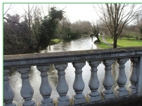
Balustrade to bridge over the River Cam
