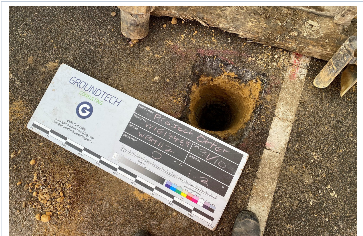
Photograph 17 – WBH112 Inspection pit
