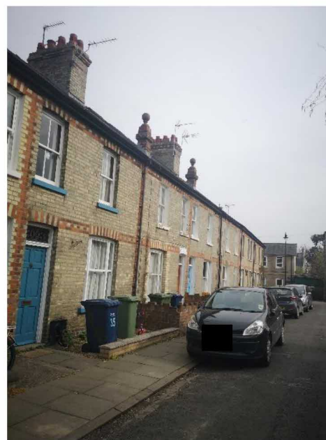
Figure 19 - View of Abbey Road, showing finial detail to No 37.
