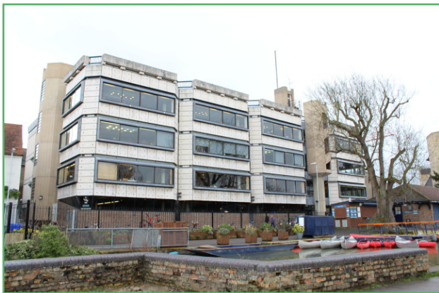
The University Centre - Grade II Listed Building
