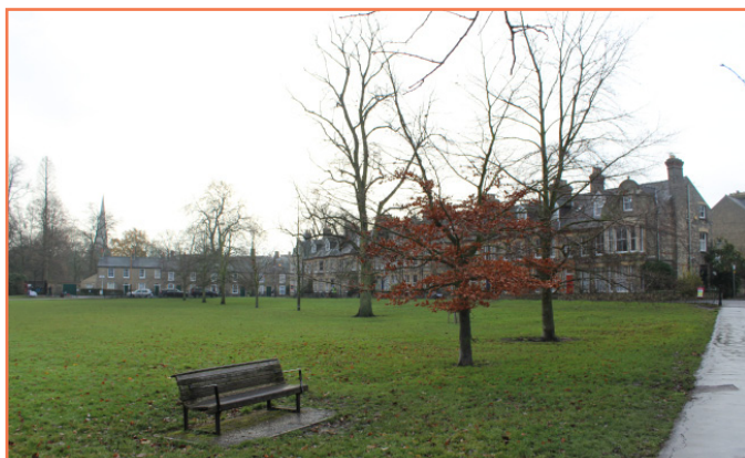
Terraced houses to Lower Park Street and Park Parade
