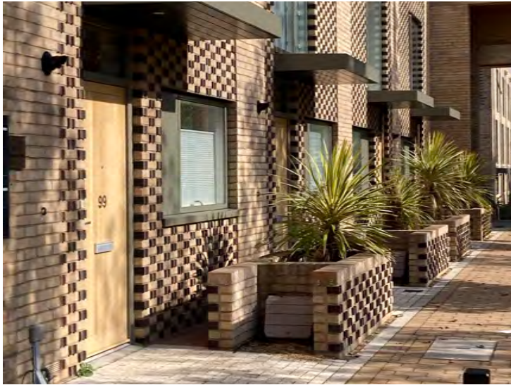
Patterned brick work expressing entrances and hiding services, Abode, Proctor Mathews
