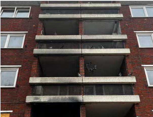
Image of a flat block deck access
