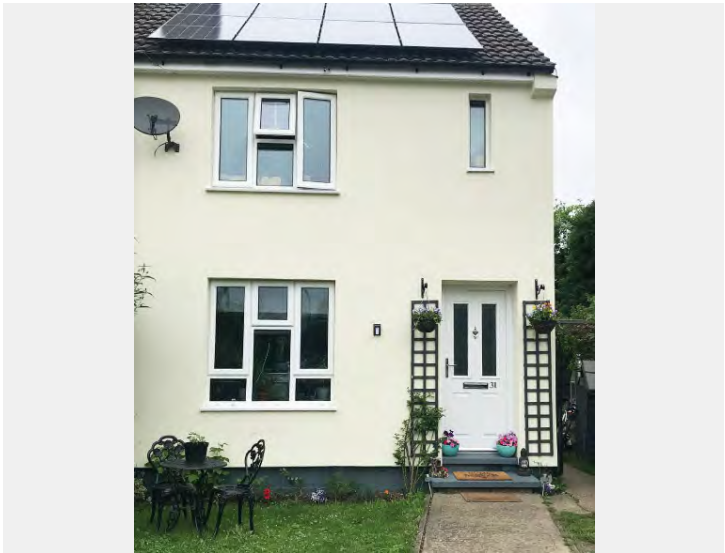
Insulated render retrofit project, Cambridge City Council
