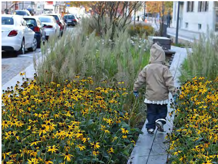
Integrating play within sustainable storm water management
