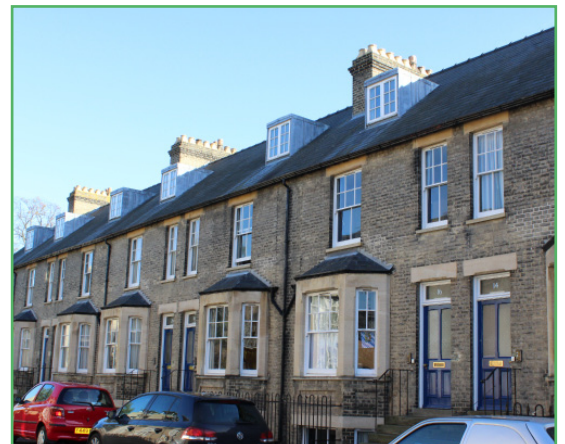
Terraces set back from the road
