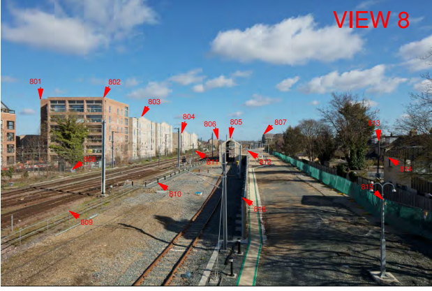
Fig 03: Survey points as highlighted by surveyor
