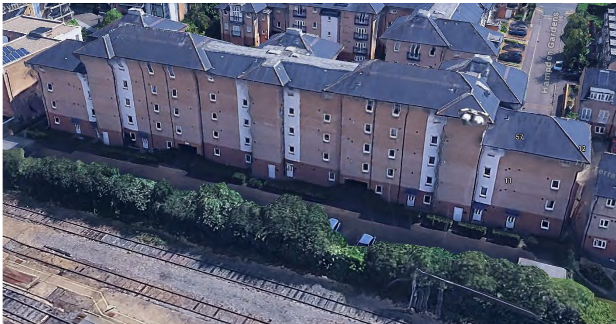
Image 1 - Aerial view of northern elevation across 55-97 Hampden Gardens
