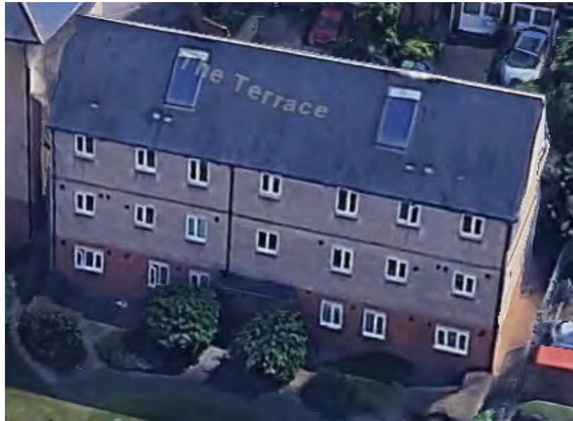
Image 1 - Aerial view of northern elevation of 11-17 The Terrace
