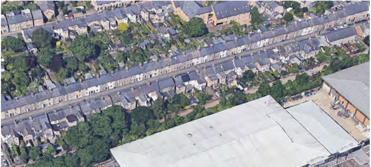
Image 1 - Aerial view of rear elevation across 2-92A York Street
