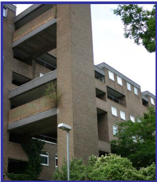
No. 18 is a white painted brick house with a low pitched roof behind a parapet. Six
