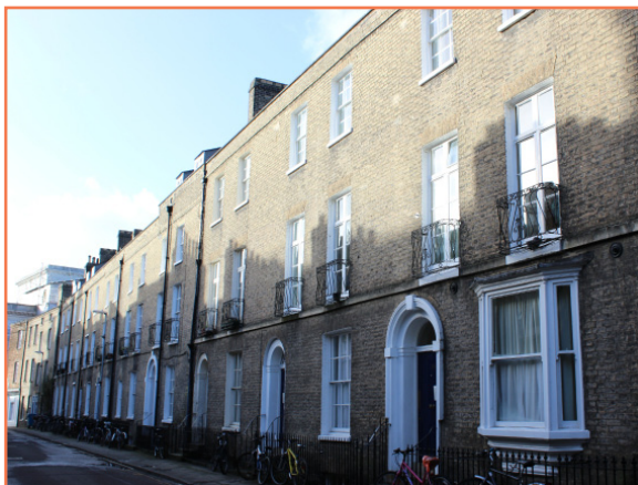
Repeated architectural features
