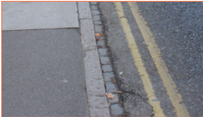
Granite kerbs and cobble setts
