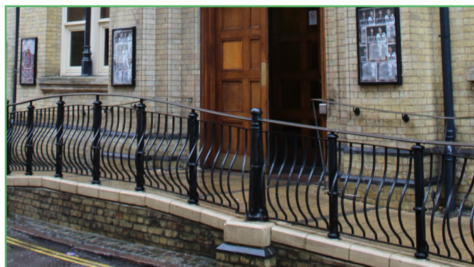
Railings to Corn Exchange ramp
