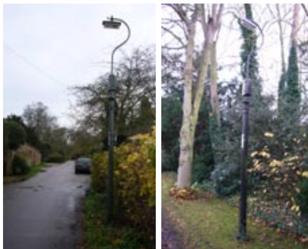
Kings Mill Lane gas standard converted to electricity (Left) Gas standard converted to electricity in Woodlands Road (Right)
