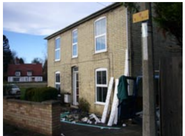
PVCu windows being installed at No.58 Woollards Lane
