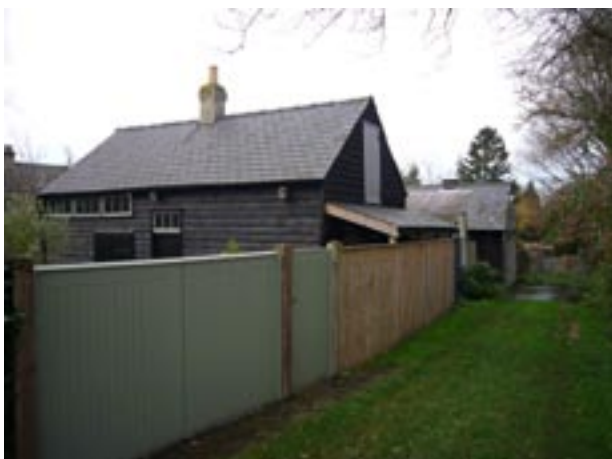
Stables and lofts at rear of Nos 35 and 37 Tunwells Lane
