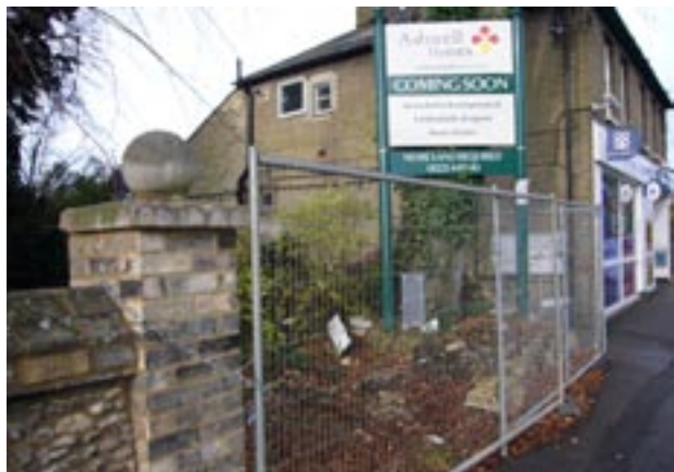
Demolished gate pier at entrance to planned housing development alongside No.76 High Street
