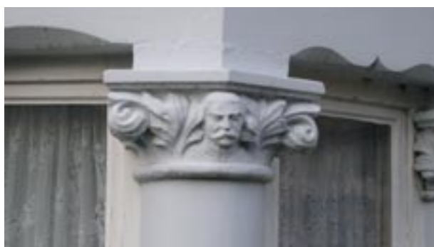
No.16 Woollards Lane (No. 1 Mow Cop Villas)
