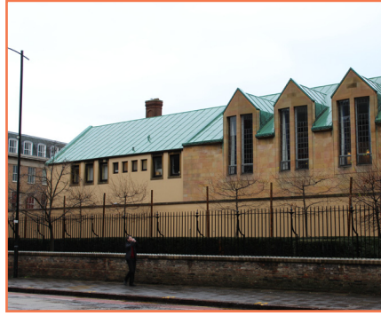
Buildings set back from the street
