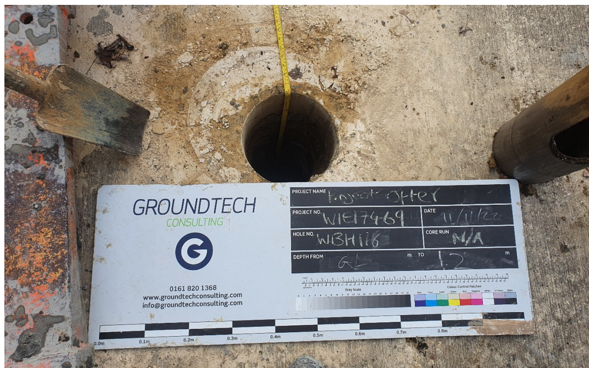
Photograph 21 – WBH116 Inspection pit
