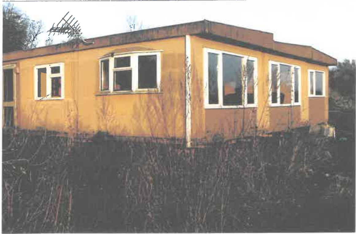
MOBILE HOMES ON SITE
