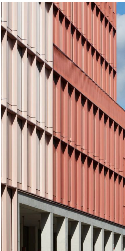
Slight tonal changes in facade materiality. R7, London, Morris+Company
