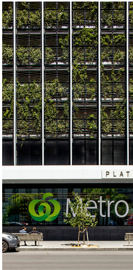
An active ground floor with car parking above. Platinum Tower, Melbourne, Squillance
