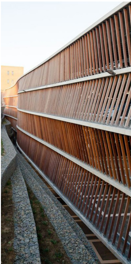
High quality and expressive car parking facade using vertical fins. Cliniques University Parking Garage, Belgium, Modulo Architects
