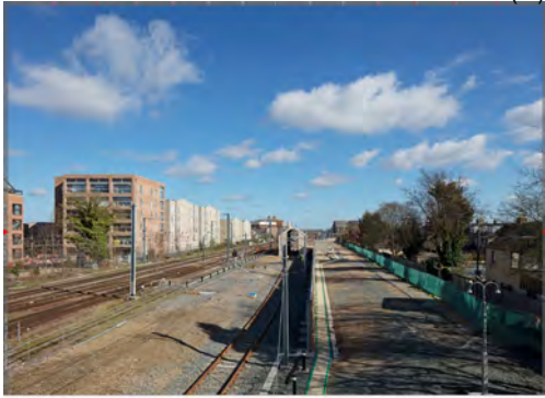
View from Mill Road Bridge (IS)
