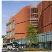
Above: Broadmarsh car park, Nottingham, Leonard Design Architects
