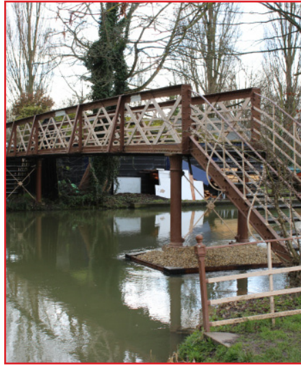
Victorian cast iron bridge
