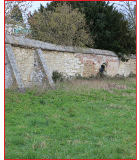
Long boundary wall to Peterhouse College
