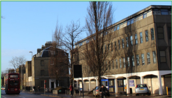
Police Station and Recency villas
