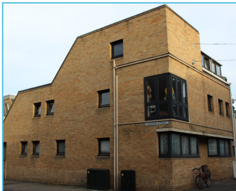
Manor Place flats
