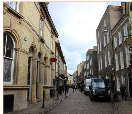
Street view looking east
