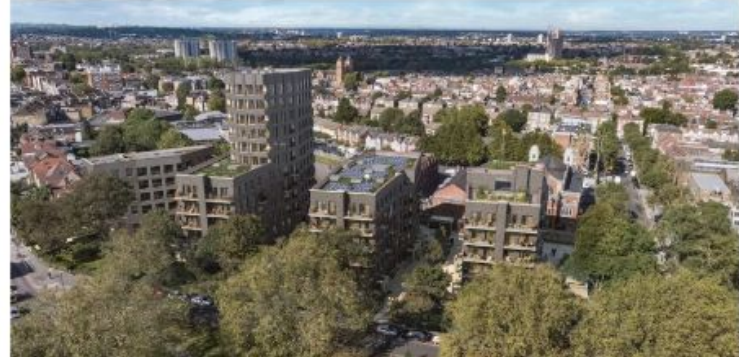
Tower Court Adam Khan Architects, Countryside Partnerships - completed in 2023
