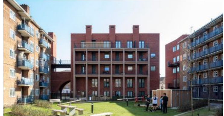
Frampton Park Henley Halebrown, Buildmore - completed in 2020
