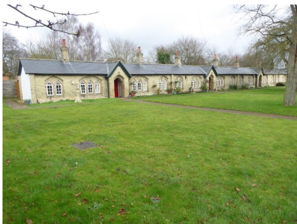
Almshouses, 23-37 Church Lane
