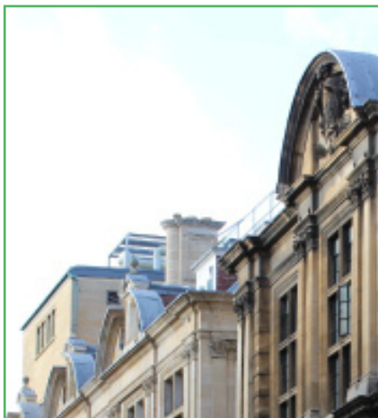
Elaborate roofline of gables and dormers
