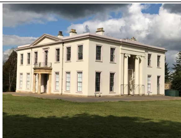
View of the Hall from the SE
