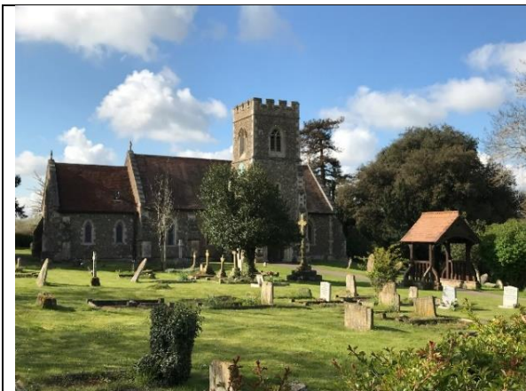
View of the church from outside St Peter's House
