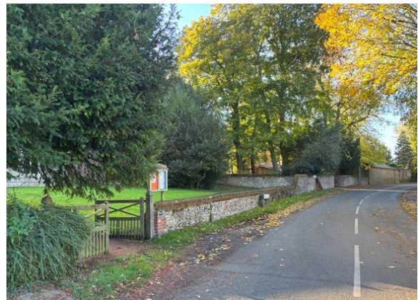
Image 15: Flint walls, Holy Trinity Church, Chishill Road
