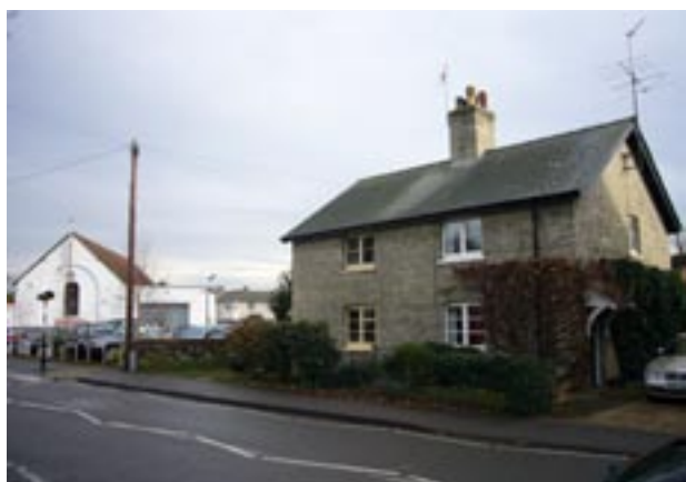
Nos. 7 and 9 Church Street
