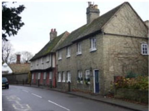
Nos. 21 and 23 Church Street
