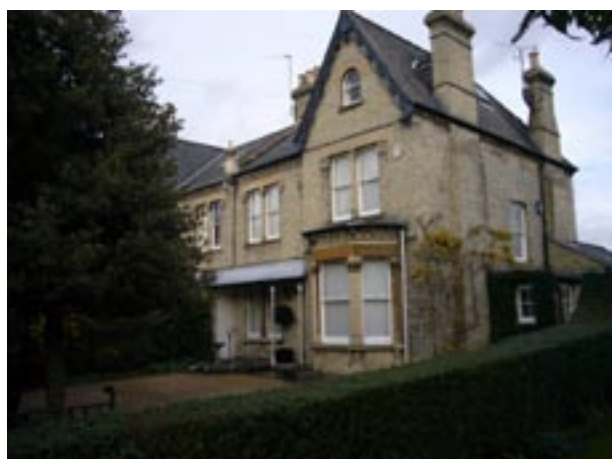
No.39 Tunwells Lane
