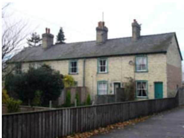
Nos 8 to 16 High Street
