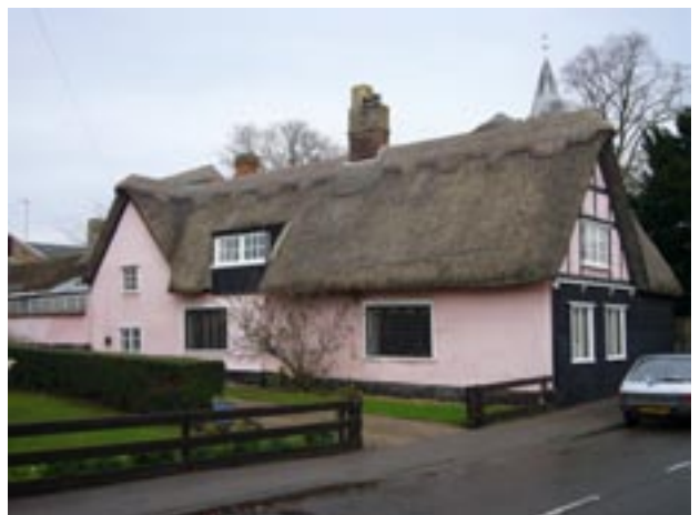
No.24 Church Street
