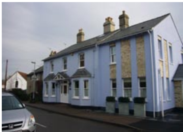
No. 11 Church Street
