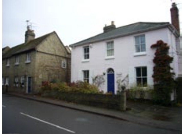
No. 25 Church street
