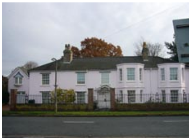
The Grove, No. 15 High Street
