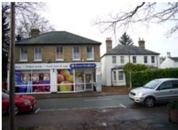
Nos. 76 (the Co-op) and 74 High Street
