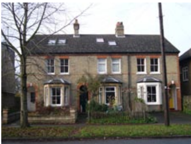
Nos. 26 to 30 High Street
