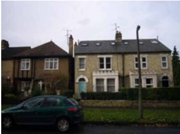
Nos. 20 to 24 High Street
