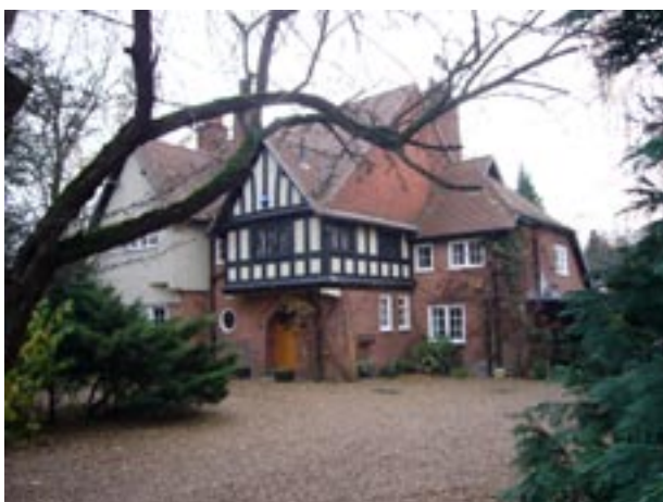
No.44 Tunwells Lane
