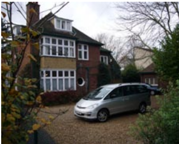
No. 38 Tunwells Lane
